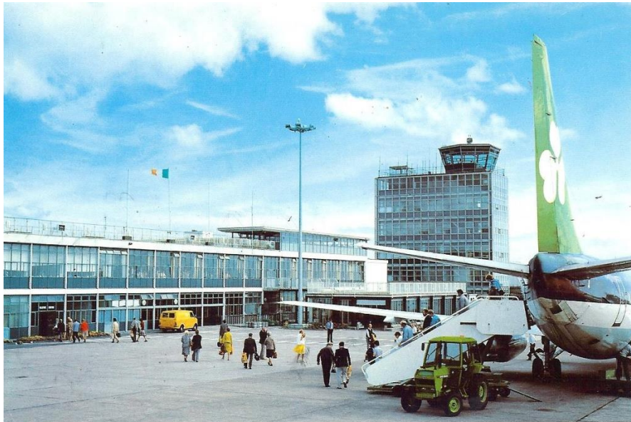
The Terminal Building, Cork Airport, Ireland.
